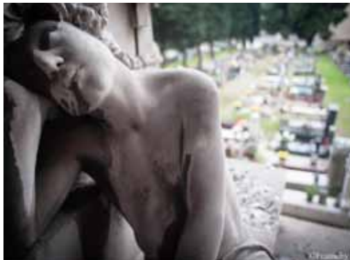
Fig. 4 Presence of "black crusts". Photo by Lucardi.
